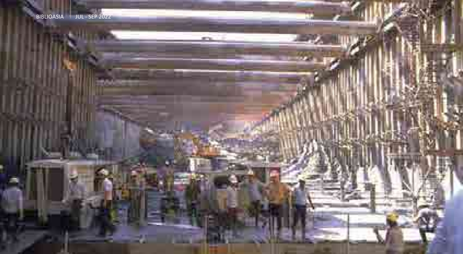
Workers constructing the underground Dhoby Ghaut MRT station, 1986. Ministry of Information and the Arts Collection, courtesy of National Archives of Singapore.
